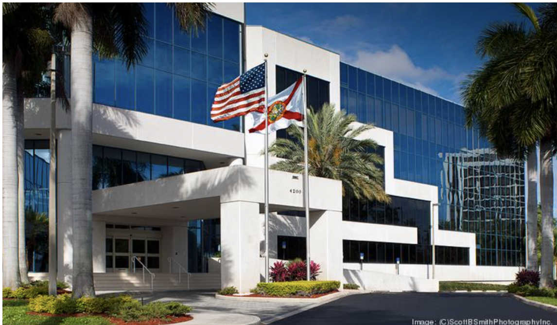
Corporate Center at the Gardens, 4200 Northcorp Parkway in Palm Beach Gardens SCOTT B. SMITH PHOTOGRAPHY, INC.
