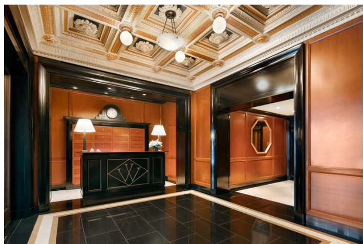
The lobby's ceiling coffers have been restored and relocated from Frank W. Woolworth's former private office on the 40th floor. Photo: Travis Mark
