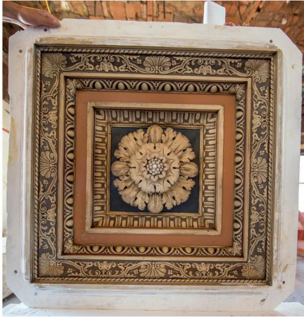
Left, one of the ornate ceiling coffers being resorted, reinforced and relocated from the 40th floor to the new residential lobby. Right, a rendering by Williams New York of the resorted ceiling coffers in the new residential lobby, which draws inspiration from the original vaulted mosaic lobby still used today by office tenants. The new lobby will have an entrance on Park Place, maple paneled walls and Crema Marfil, Indus Gold and Belgian Black marble floors.
